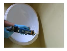
1. Apply a small bead of silicone around the top edge of the washbasin, making sure to follow the directions on the label.
