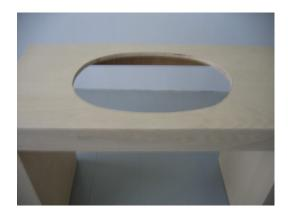
Use a template to draw the cutout line on the countertop. If there is no template provided, then place the bowl upside down on the countertop and trace around the outside edge. Then draw a second line 3/4" inside that line, and use this as your cut line. Then perform the cutout
