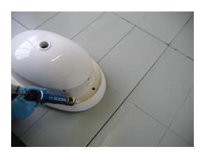
2. If the faucet is to be installed onto the actual sink, then install the faucet first. Otherwise just turn the sink upside down and apply a small bead of silicone on the underside of the molded lip.
